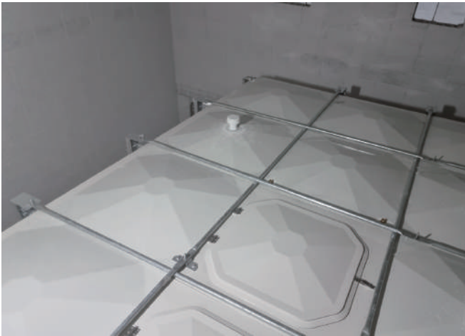
Steel poles on roof
