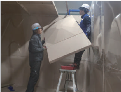
Roof Panel Assembly
