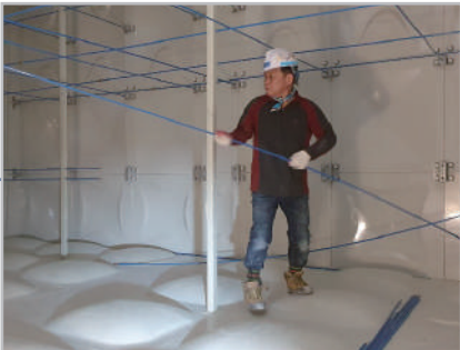
Roof Support, Tie-rod, Internal Ladder Assembly
