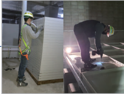
Attach Nozzles & Sealing Tape
