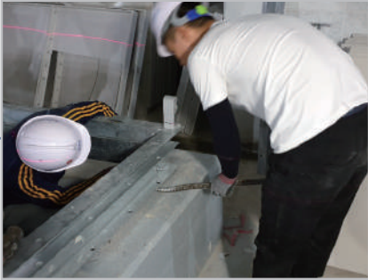
Install Skid Steel Base
