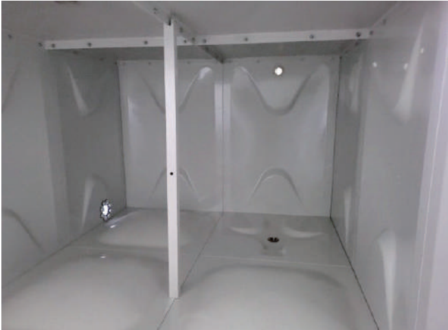
Tank inside (No Tie-rods)
